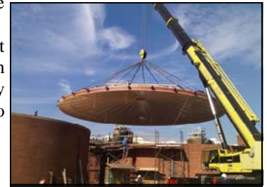
Installation of New Digester Cover at the Yonkers WWTP
