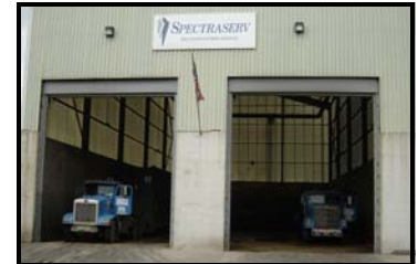
Spectraserv Transfer Facility
